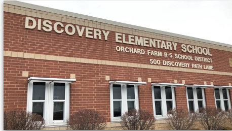
Discovery Elementary (8 classroom addition)
