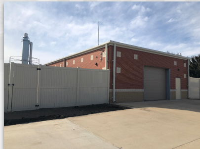
Water Treatment Facility
